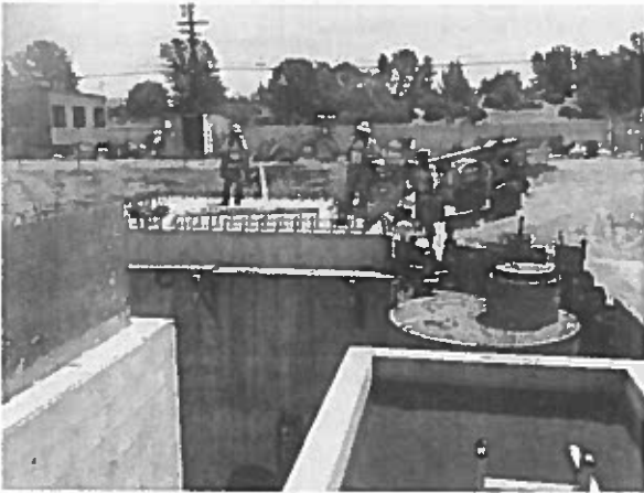
The Contractor assembles formwork for Wet Well SOG.
