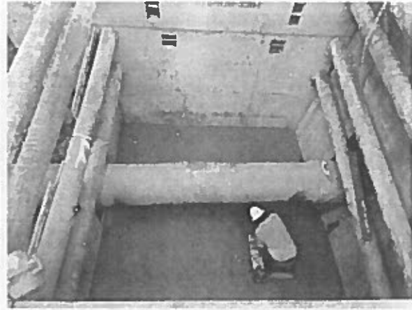
The Contractor smooths out concrete pad after concrete pour is performed.
