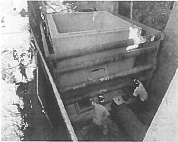
The Contractor installs precast concrete sections for the Pond Meter Vault
