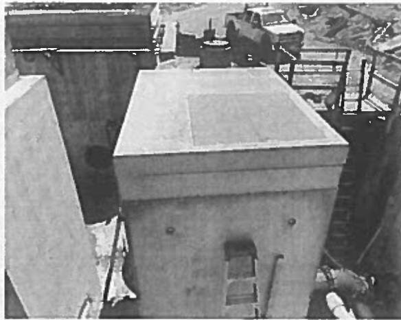
Precast Concrete lids are temporarily placed over both Diversion Boxes.
