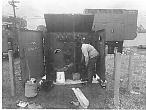
PG&E installs and energizes the transformer and switchgear.
