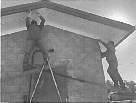
The Contractor paints roof soffit for electrical building.
