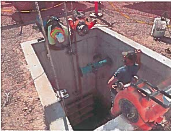
Contractor installs slide gate actuators.
