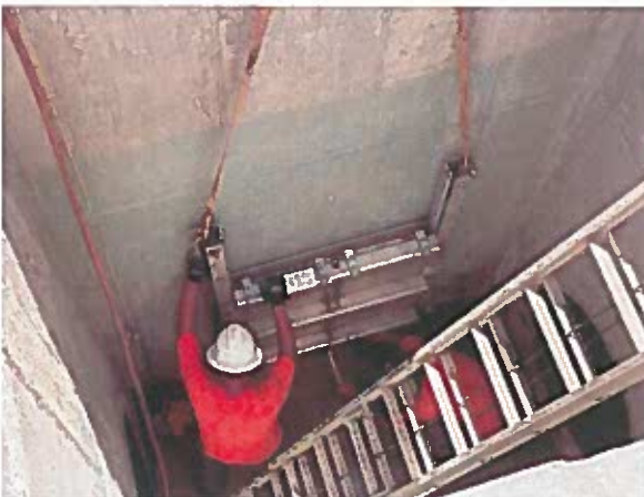
The Contractor installs a slide gate at Diversion Box 1.
