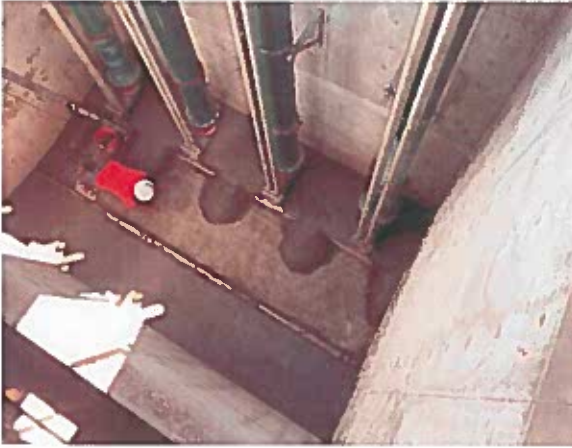
Contractor places grout at bottom of wet well.
