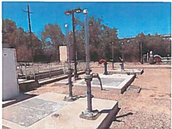
Diversion box lids are replaced and actuator hand cranks are installed.
