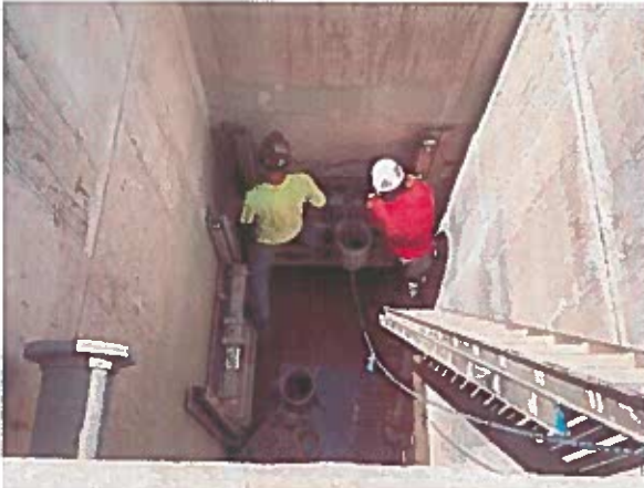
The Contractor installs and grouts slide gates in Diversion Box 2.
