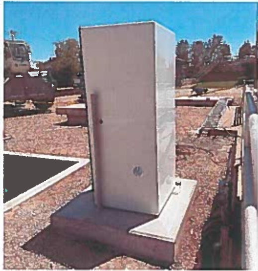
The manning sampler is installed.
